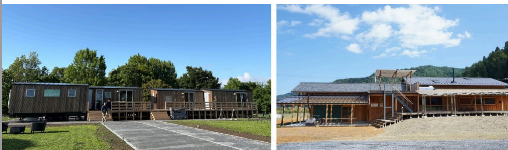
Exterior views of the two most recently opened Nagisa-no-Koban beach facilities – Nagisa-no-Koban Toda Aya Lake Base (left) and Nagisa-no-Koban Ishinomaki Moriumius Marine & Food (right)
